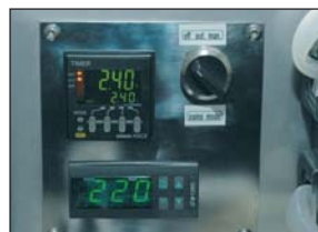
Electronic check of weld temperature, filling timer and AUTO switch
